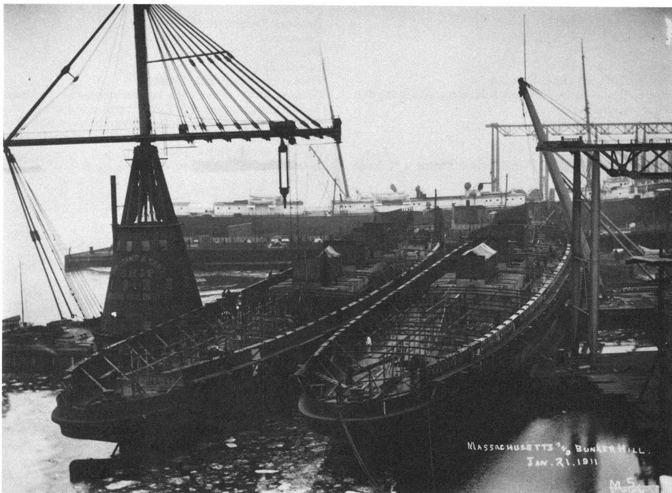
Conversion of Massachusetts and Bunker Hill (Hulls 342, 343) into passenger steamers, photograph by J. S. Huse, 1911. FI Collection at PMM (L90.43.X34).
