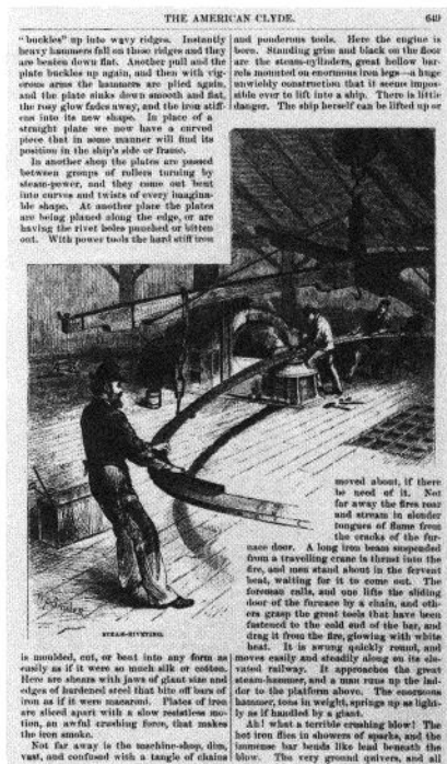
These engravings accompanied an article on the Delaware Valley's iron shipbuilding innovators in Harper's New Monthly Magazine (1878). Stages in the production process included (left to right): bending stem bar, perforating angle-iron, and steam riveting. Van Pelt Library, University of Pennsylvania.
