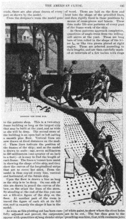
These engravings accompanied an article on the Delaware Valley's iron shipbuilding innovators in Harper's New Monthly Magazine (1878). Stages in the production process included (left to right): bending stem bar, perforating angle-iron, and steam riveting. Van Pelt Library, University of Pennsylvania.
